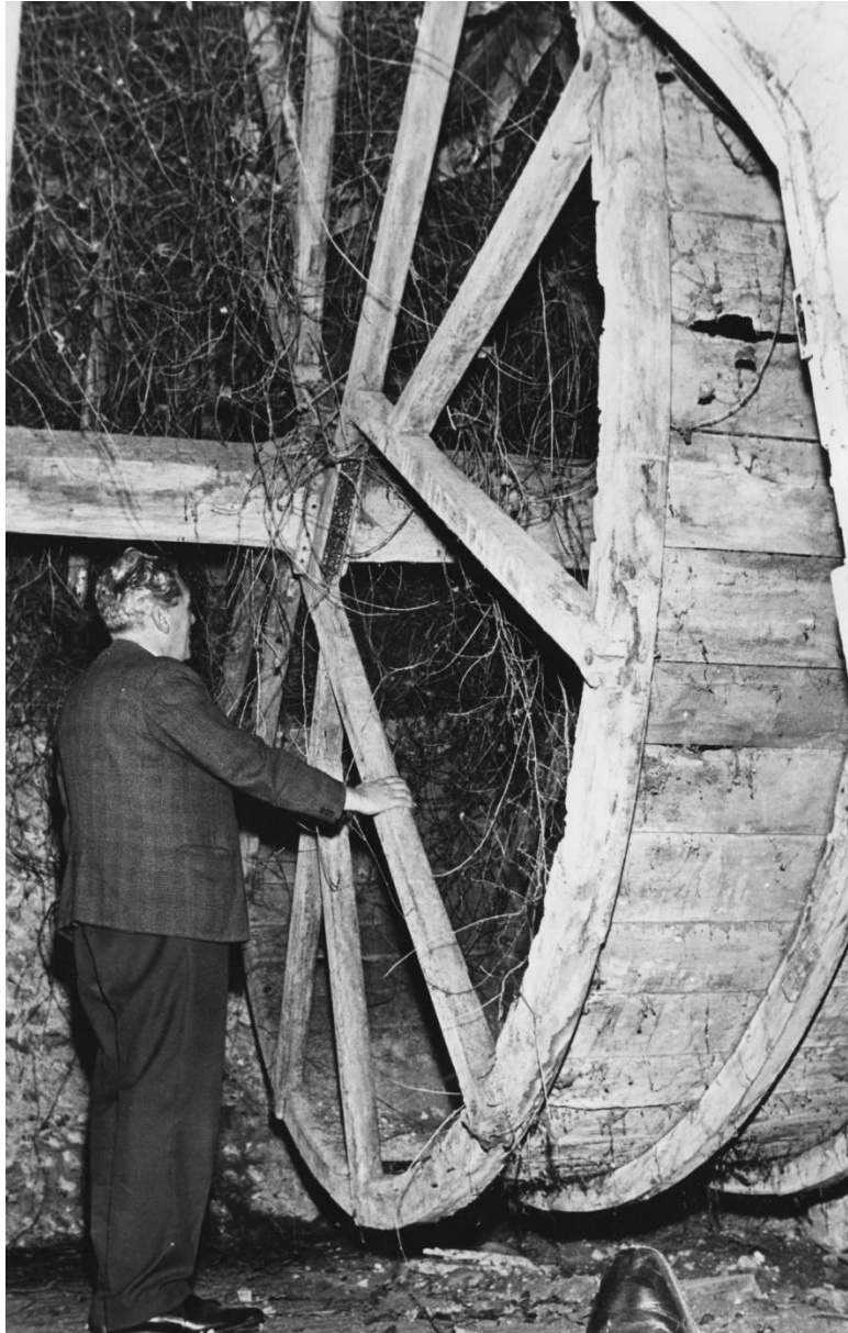
Figure 24: Inspection of the donkey wheel prior to repair 1968 (Source: SPS).
