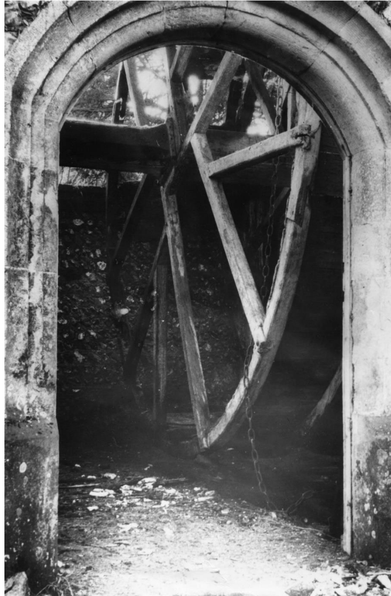
Figure 25: The roof of the well house removed during repairs 1970 (Source: SPS).
