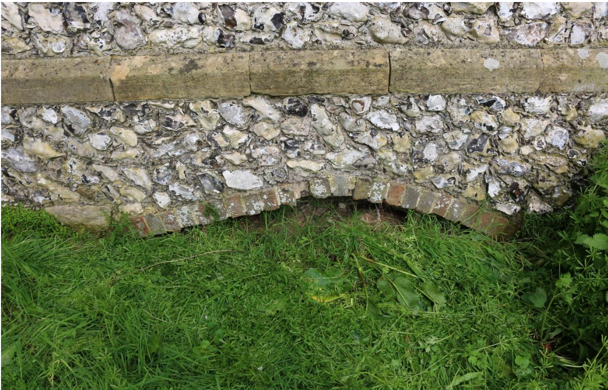
E. Shallow brick arch - east elevation.
