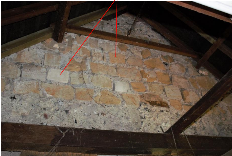
Dressed sandstone reused in gable repair
