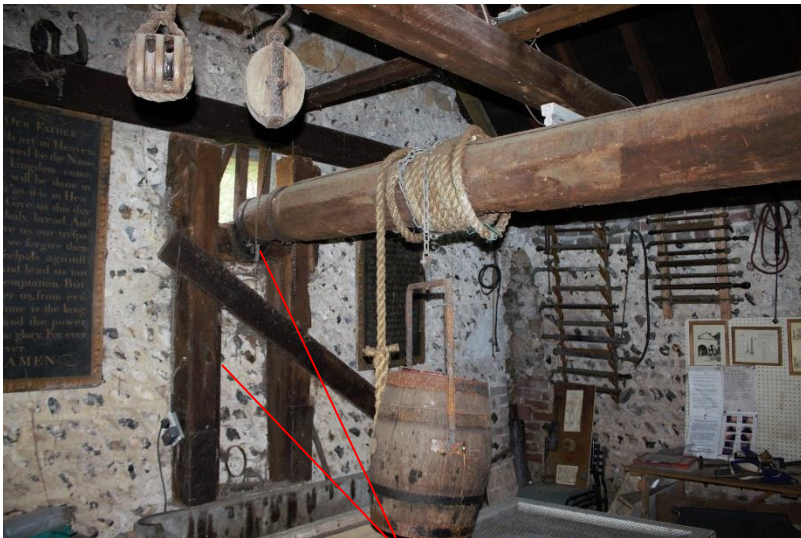
Oak wheel shaft with ironwork bracketing and posts with mortise holes
