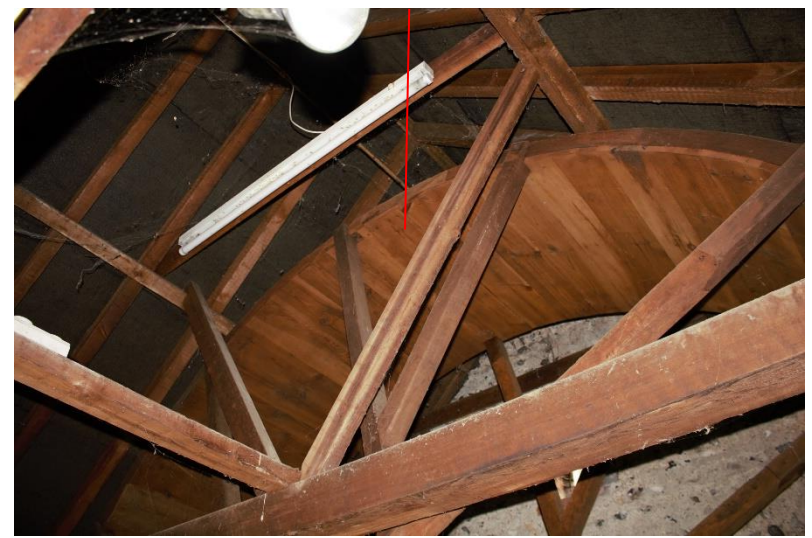
Modern replacement wheel slats
