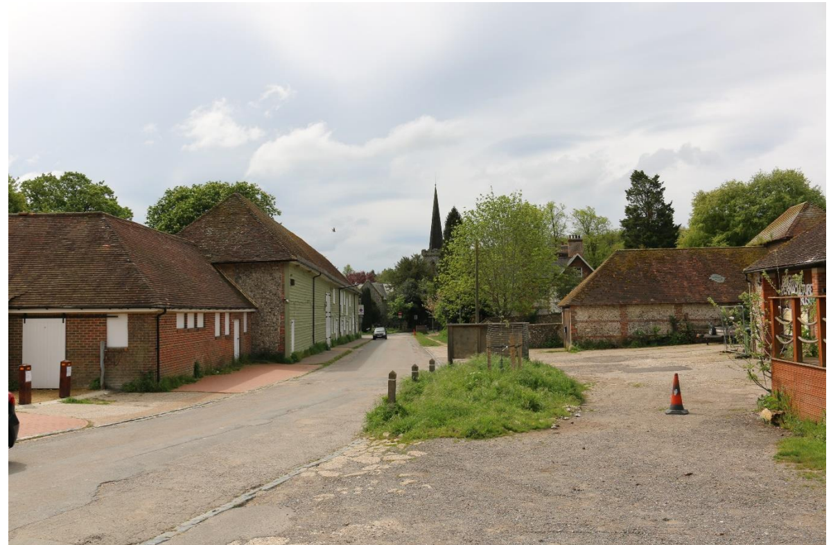
D. View looking south from Home Farm, showing farm buildings including Home Farm Barn.
