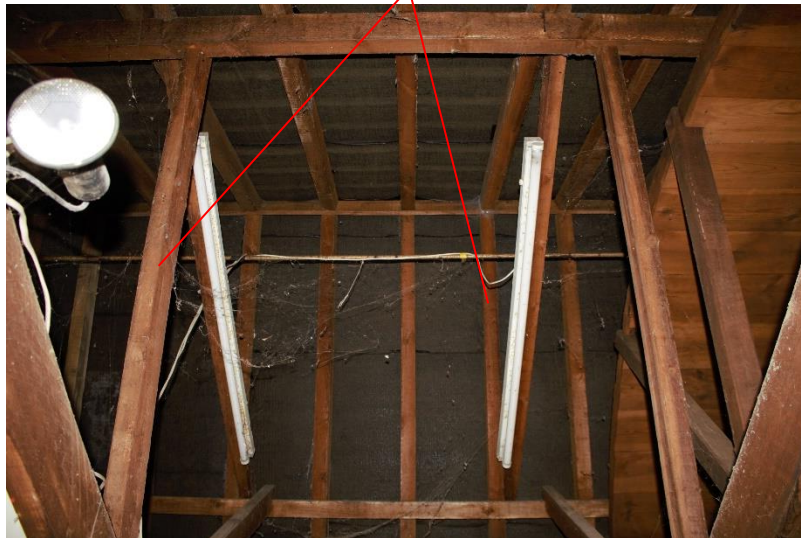
Machine cut timber roof frame
