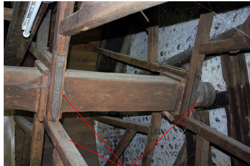
Clasp-armed wheel spokes, ironwork reinforcement and mortise and tenon joints
